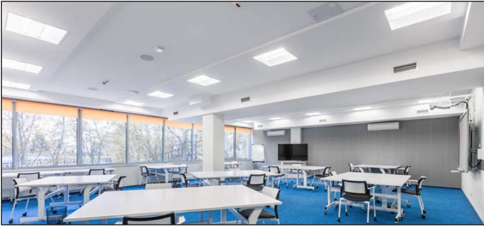
The Troffer Retrofit center-basket design includes a diffused lens that delivers soft, even ambient light.
