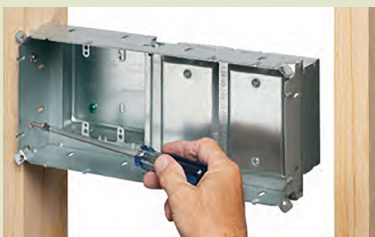
Attach box to stud using #6 screws. Pull wires.
